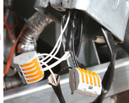
Figure 24: Wago connectors
